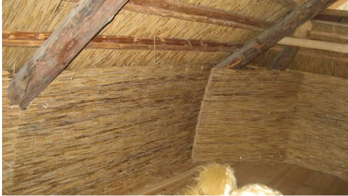
Figure 3.43 Properly insulated attic (Photo: S. Söber)
