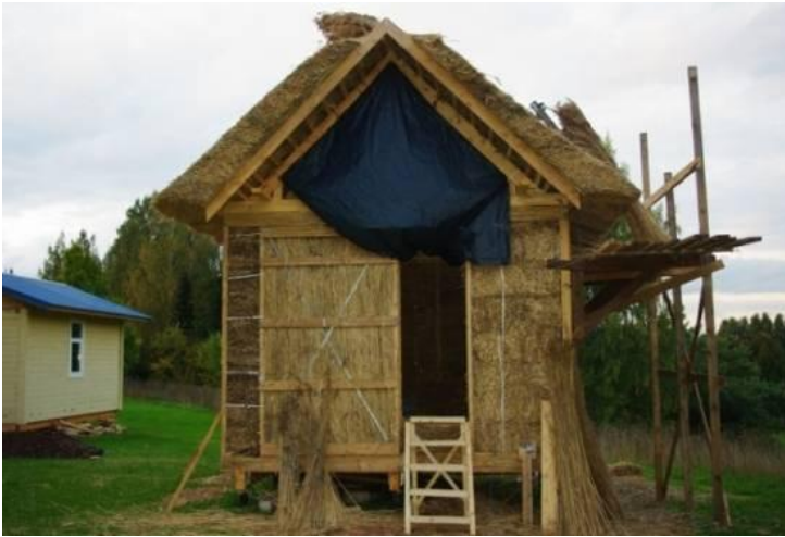
Figure 3.21 a Wall VS-1 (vertically laid reed wall)
