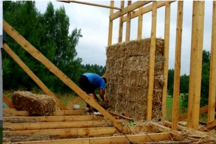
Figure 3.21 d Wall VS-4 (reed block wall)
