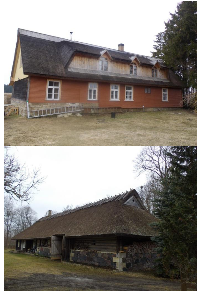
Figure 3.38 Farms studied. Upper: thatched roof with ridge covered with aspen boards and lower: the hip roof with vey holes and traditionally reinforced ridge (Photos: S. Sõber)
