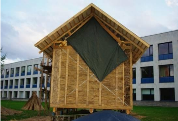
Figure 3.21 c Wall VS-3 (reed panel wall)
