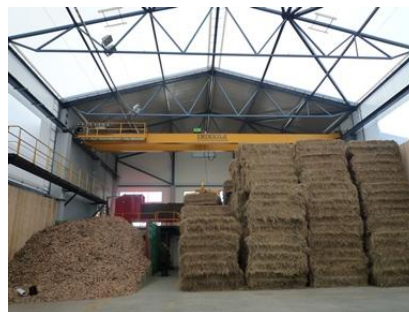
Figure 5.13 Storing of large square bales in Lihula (Estonia) boiler house storage (Photo: Ü. Kask)
