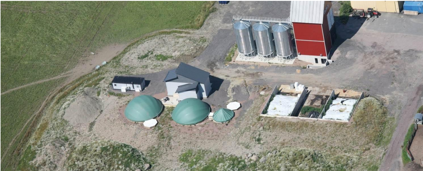
Figure 6.6. The biogas plant at Livia College
