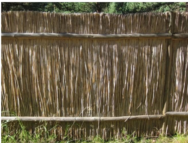
Figure 7.1 Fence made of common reed covers the view and protects well from the wind and sunlight. (Photo: A. Hemmi)
