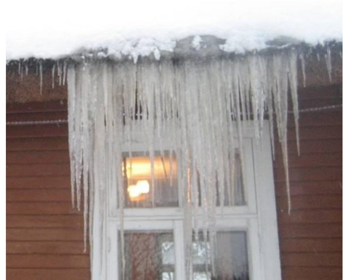
Figure 3.44 Icicles on the eaves of thatched roof (Photo: S. Söber)
