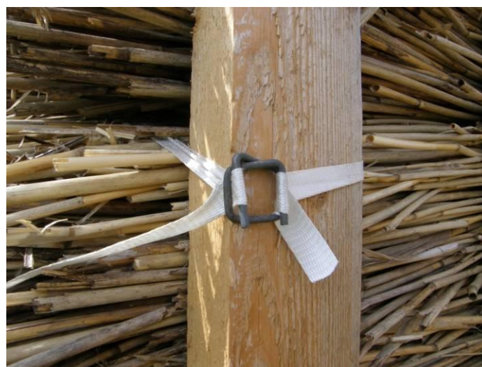
Figure 3.23 Fixing of loose reed with plastic strings (wall VS-2)
