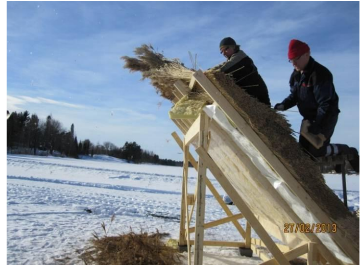
Figure 3.33 Petri Iivonen levelling the eave's end with a specific tool.
