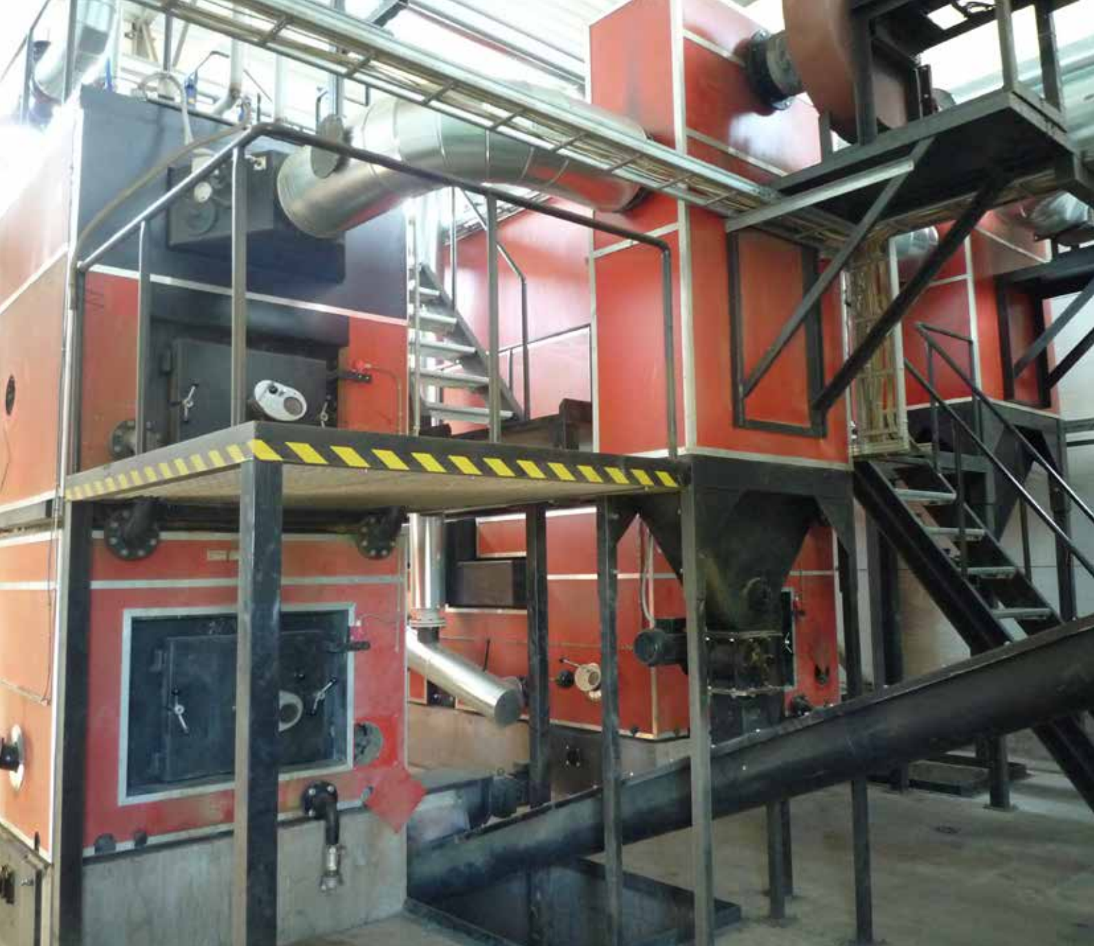
AS-i Tootsi Turvas katlamaja Lavassaares. AS Tootsi Turvas boiler house in Lavassaare borough.
