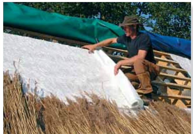
A fireproof fabric is laid out above the timber and below the reed. Photo: Carlo F. Christensen.
