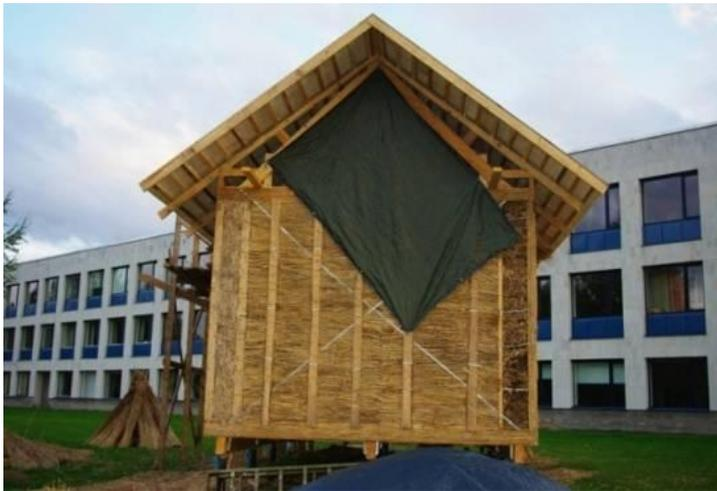
**Figure 3.2. c** Wall VS-3 (reed panel wall)
