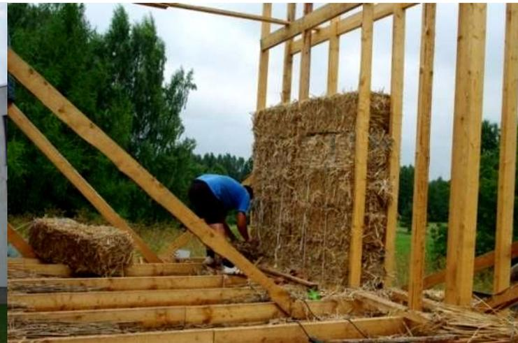
**Figure 3.2. d** Wall VS-4 (reed block wall)
