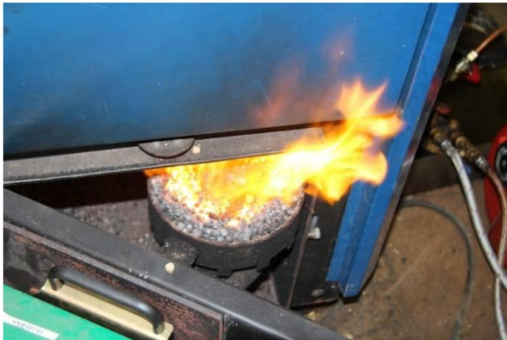
**Figure 4.13.** Pellet burner BioLine 25 (Sweden) (Photo: Ü. Kask)
