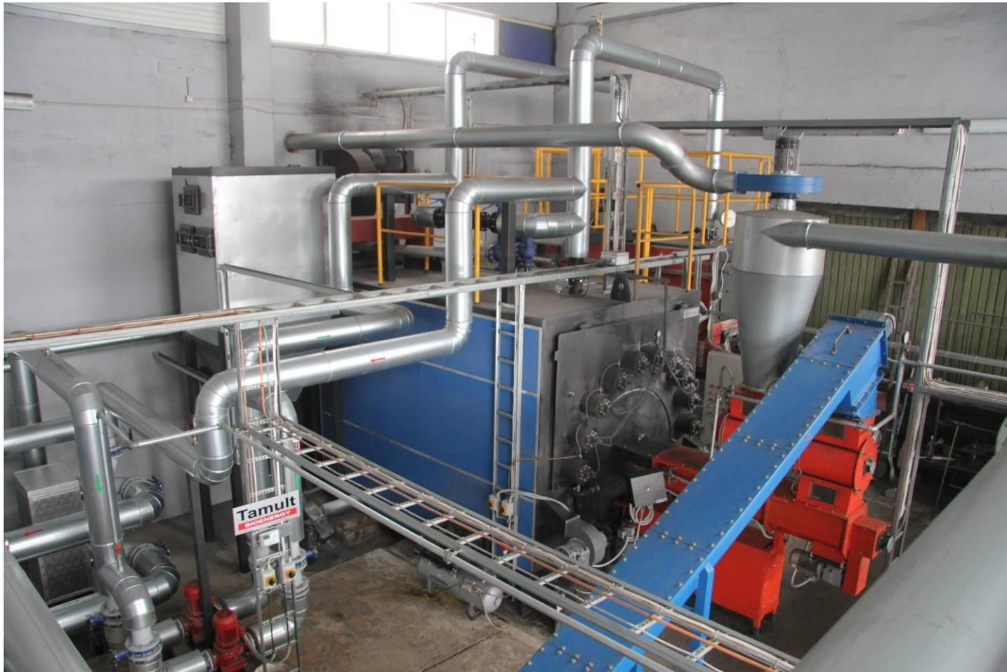
**Figure 4.9.** Danstoker biomass boiler at Lihula Boiler House (Photo: Ü. Kask)
