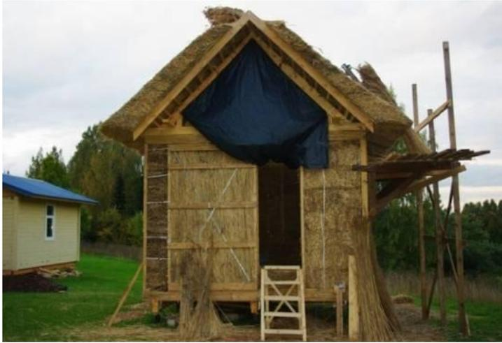
**Figure 3.2. a** Wall VS-1 (vertically laid reed wall)
