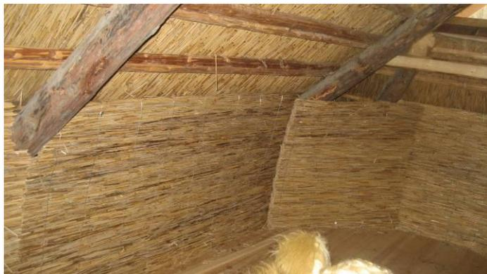
**Figure 3.43.** Properly insulated attic (Photo: S. Söber)
