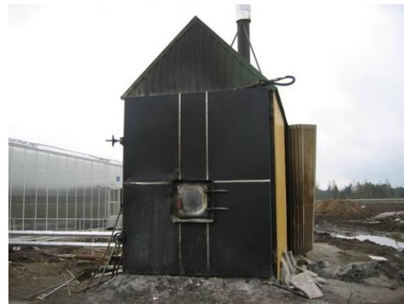
**Figure 4.6.** Boiler for burning round and square grass and straw bales (Photo: Ü. Kask)
