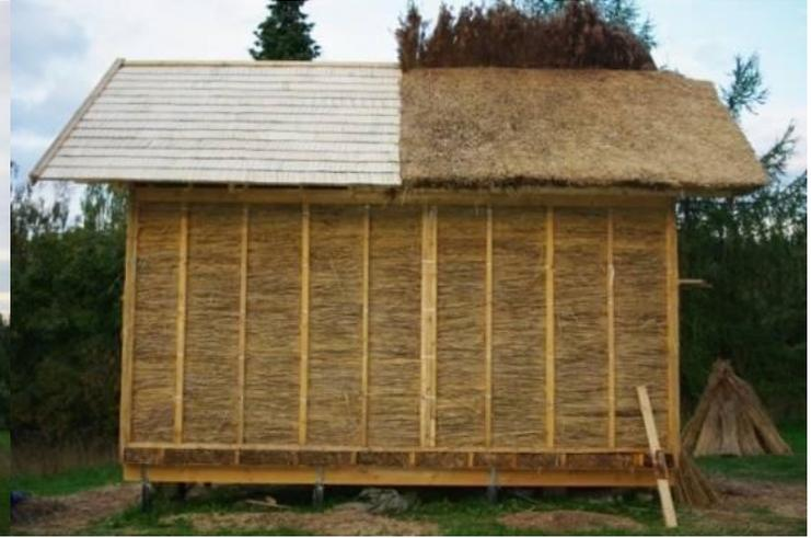
**Figure 3.2. b** Wall VS-2 (horizontally laid reed wall)
